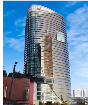
The Gardens South Tower Value: RM398 mil
