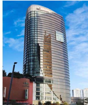
The Gardens South Tower Value: RM396 mil
