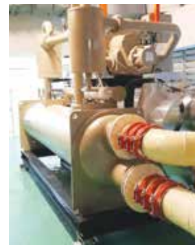
Replacement of chiller at G Tower
