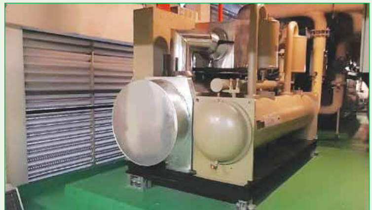
Replacement of new chiller to improve energy efficiency at G Tower
